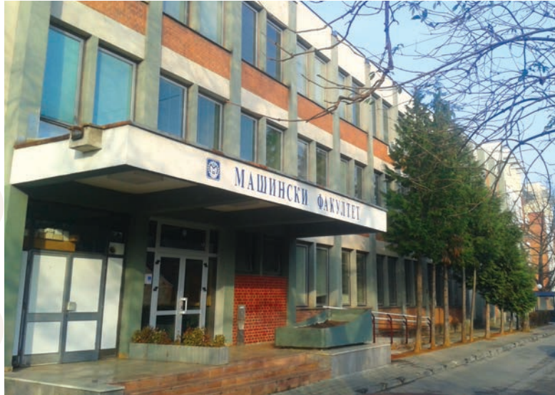
The Faculty of Mechanical Engineering in Banja Luka
